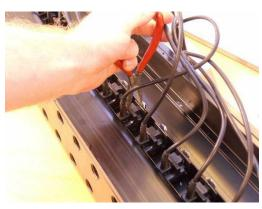
2. Release the metal clips manually or with a small plier.
